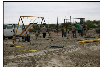
installing El Charco playground
